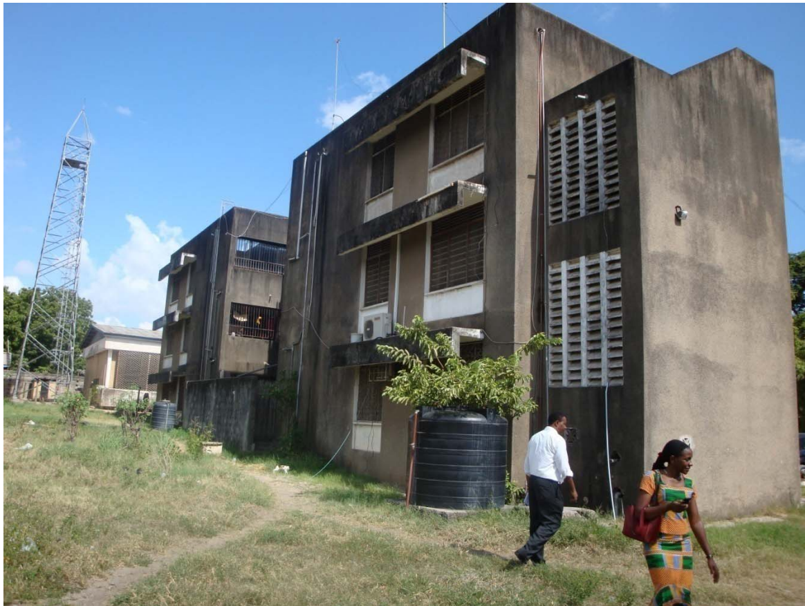
Figure 4.1: Existing Building in PPRA's Plot at Kurasini
